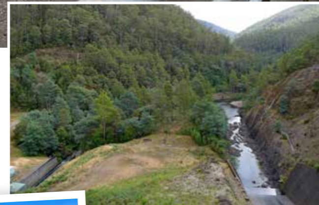
Start of the Mersey River from Parangana Dam
