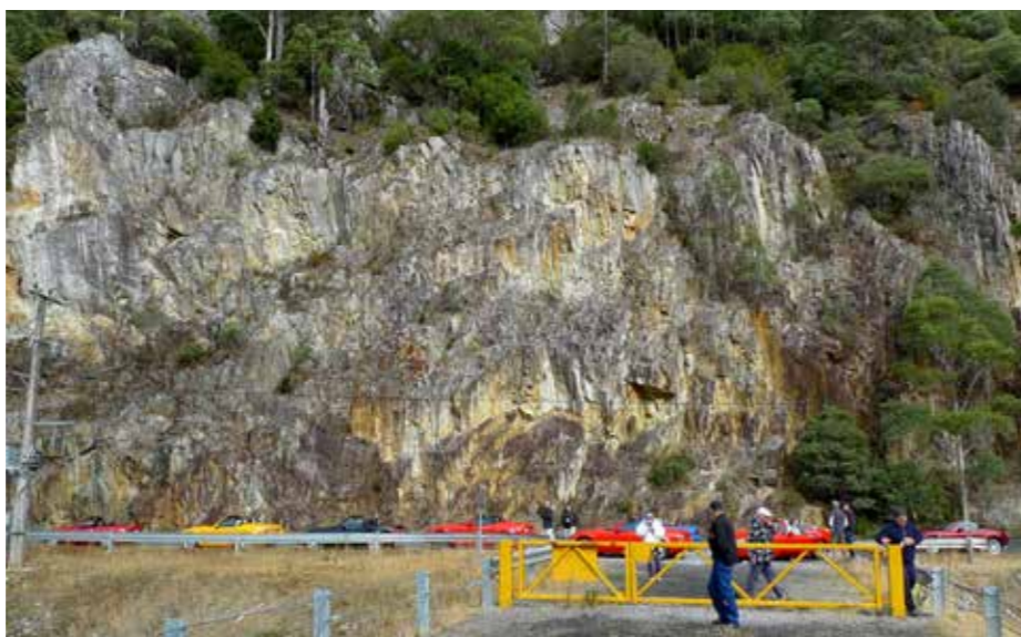
Parangana Dam ... does walking the dam count as another bridge?
